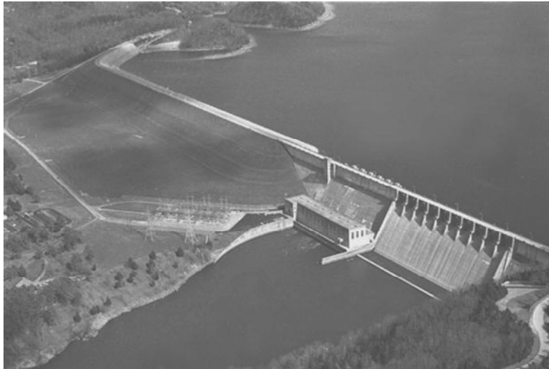
Wolf Creek Dam (USACE Photo)
